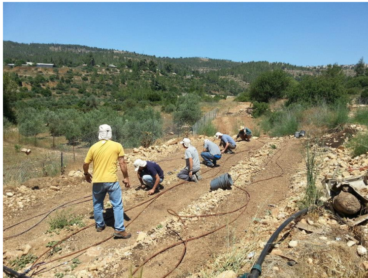
Netafim volunteers install a drip irrigation system at Beit Zayit
